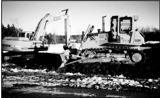
Grading the location of the new farmhouse
