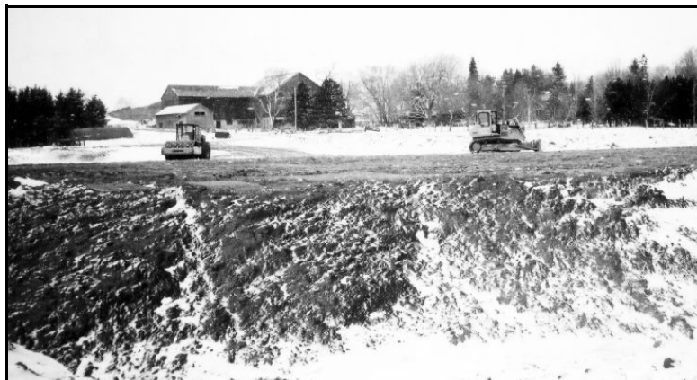
Construction site is being prepared
